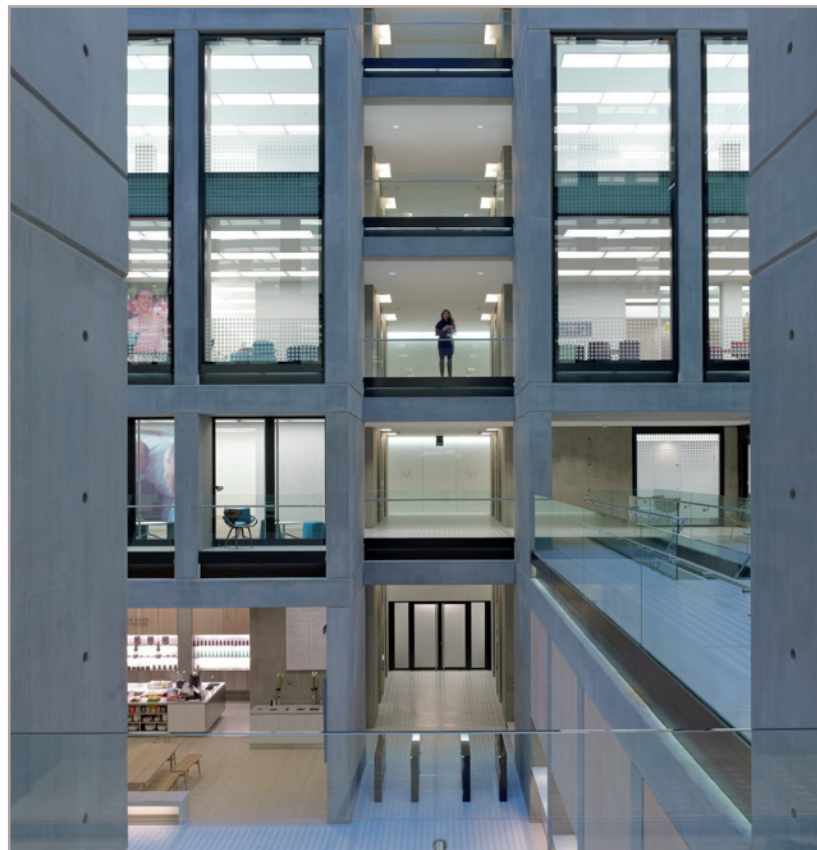
The Angel Building, London used a concrete mix containing 40 per cent fly ash replacement, which helped to achieve its dark grey finish. Image courtesy of AHMM Architects.
