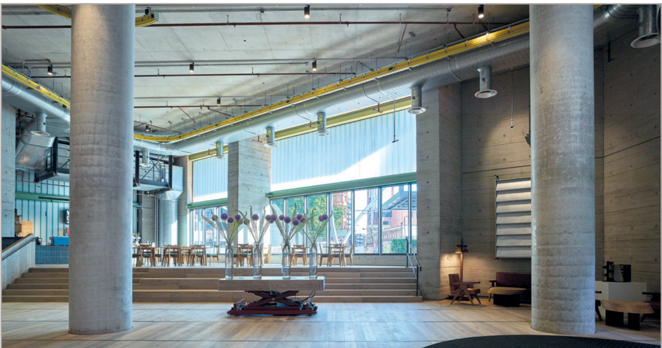
White Collar Factory, London is a BREEAM 'Outstanding' 17-storey office building that has extensive exposed concrete throughout. This provides the thermal mass that's intrinsic to its passive cooling strategy. Image © Timothy Soar
